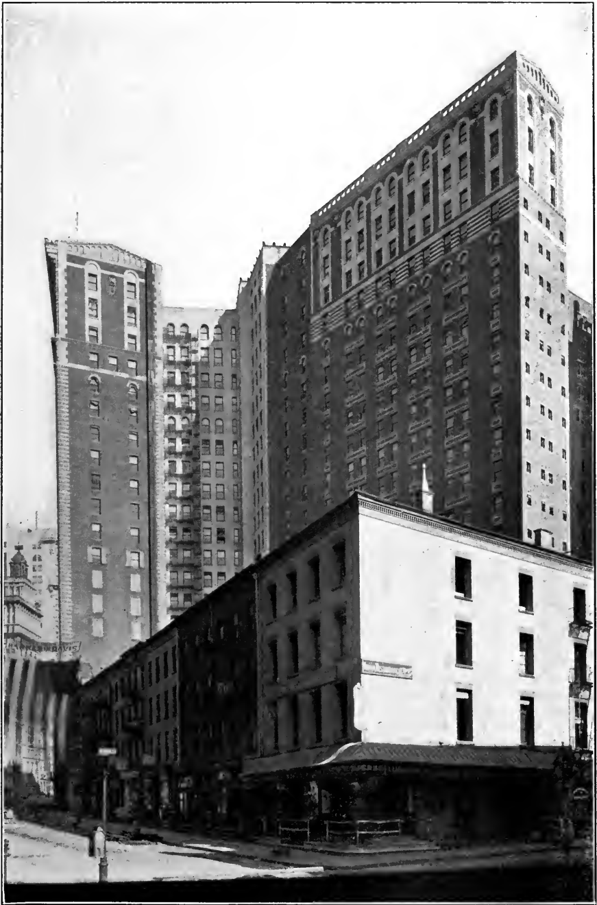
FIG. 3. THE REAR OF THE BROAD-EXCHANGE BUILDING.
